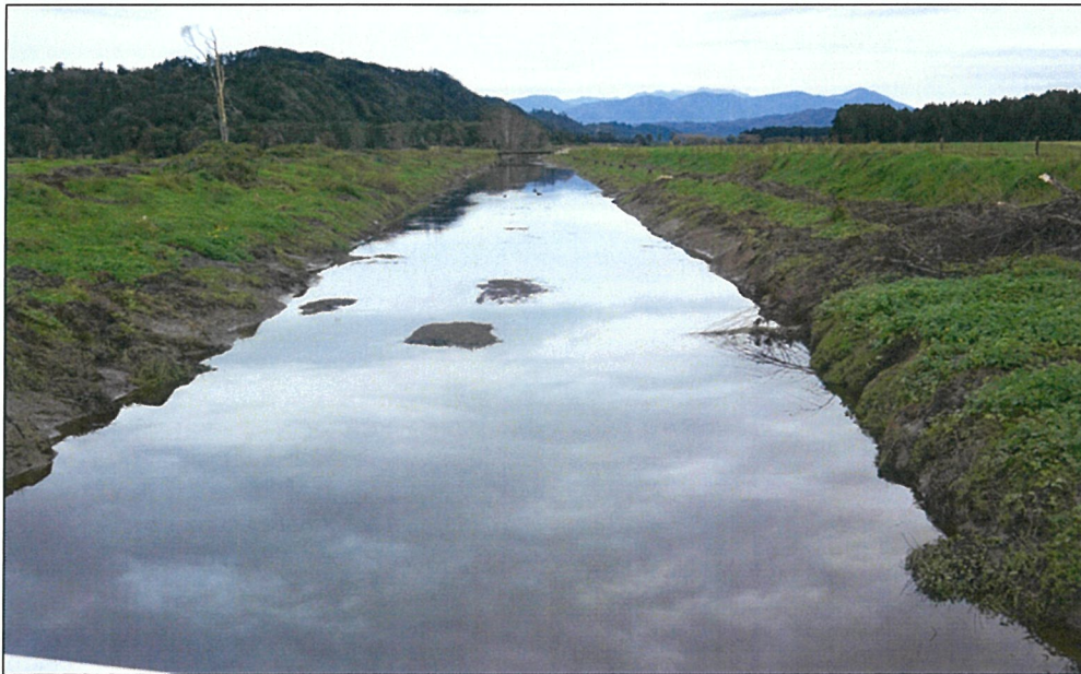
Contour channel, looking upstream following clean-out.
