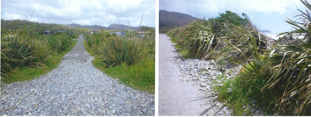
Figure 3-2: Continued overwash deposits onto Morpeth St (left) and Beach Rd near Statham St (right). [Credit: M. Hicks].
