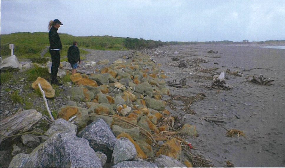
Figure 3-2: Rock extension south of the carpark to protect the Lagoon Cut entrance. [Credit: M. Hicks, 21/11/2017].
