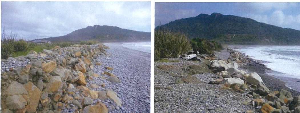
Figure 3-4: Continued beach retreat against rock berm (left) and along the entire foreshore (right). [Credit: M. Hicks].
