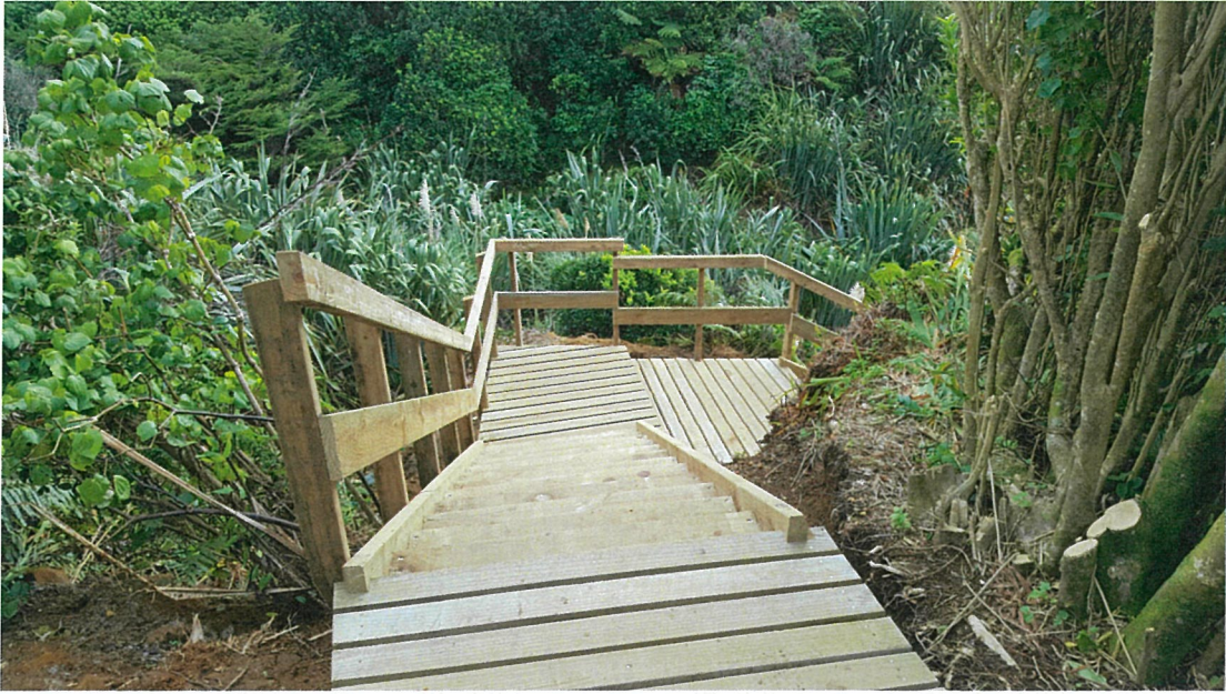
Photograph 3: Wooden staircase installed down to the beach replacing the previous arrangement
